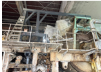
Hood support structure (in grey), along with jacking arrangements
