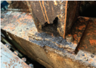
Column corrosion
