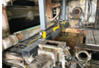
Hood support structure (in grey), along with jacking arrangements
